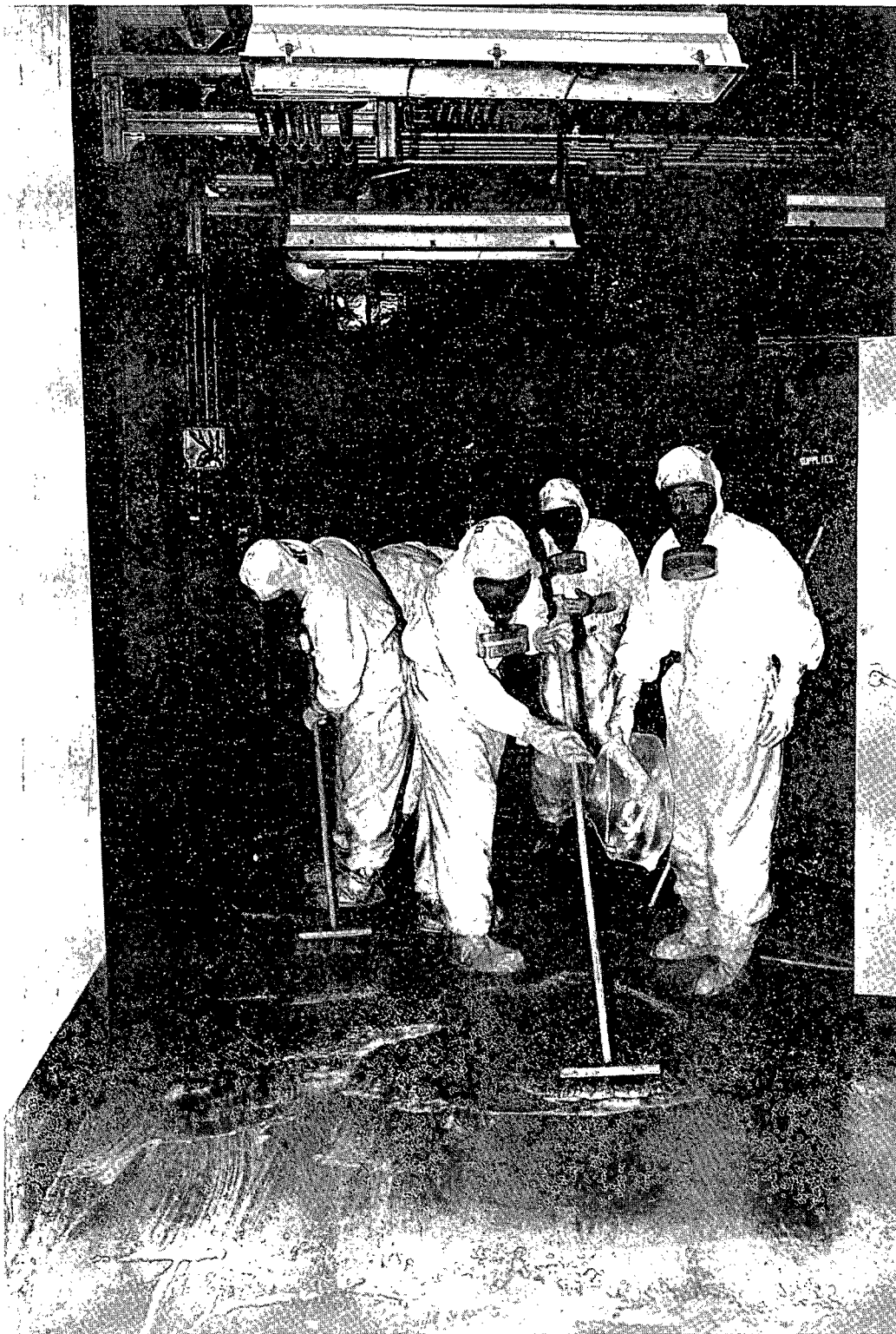
Figure 5.1. Wet Mopping of TMI-2 Auxiliary Building. Wet mopping is one technique used to decontaminate portions of the Auxiliary Building. Workers are shown wearing special clothing and breathing apparatus for protection from radioactive contamination. (Official TMI Photo)
